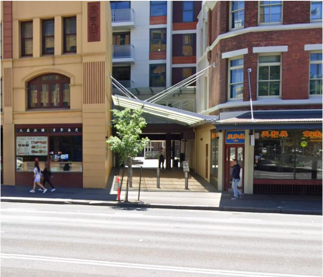
Figure 2 Arcade from Broadway sag point through buildings and Plaza towards Blackwattle Lane
